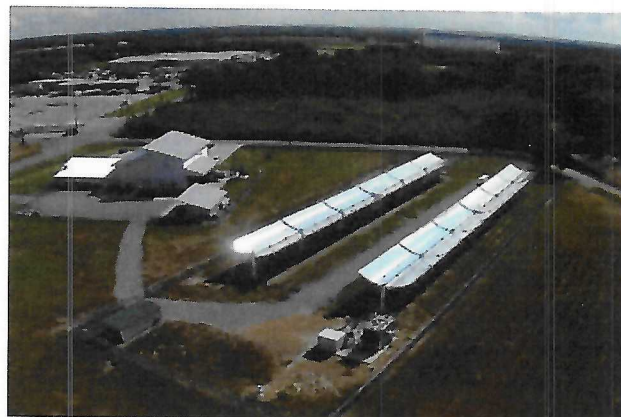
Above: The Cleco Alternative Energy Center in Crowley, Louisiana. Note the large parabolic mirrors of the concentrating solar-thermal testbed and the technology-assessment building, which houses a complete analytical laboratory, as well as the technology-assessment pilot area, which houses the gasifier and torrefaction units. Right: Growing microalgae culturing in the laboratory for both CO 2 capture and conversion into value-added chemicals.
